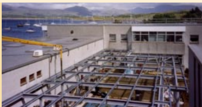
Fig 31 The new Data Warehouse building under construction within the inner quadrangle of the Laboratory.
