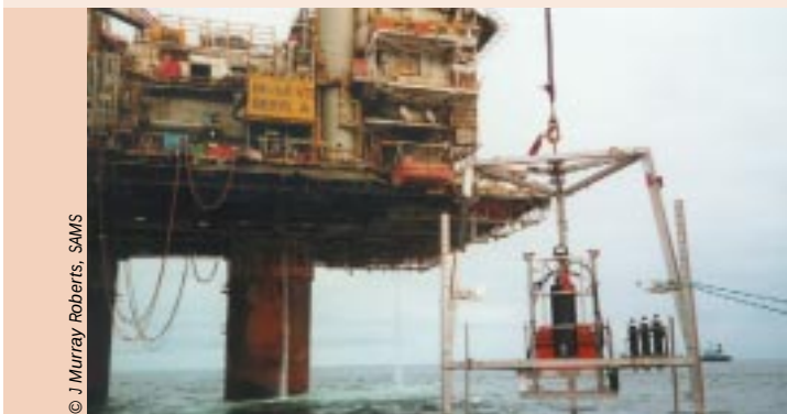
Fig. 51 DML lander being deployed adjacent to the Beryl Alpha production platform
